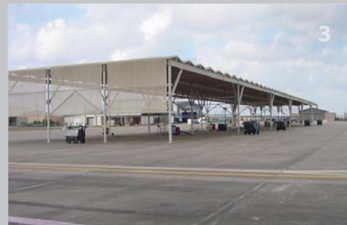
1. Apron Replacement, Ellington Field, TX
